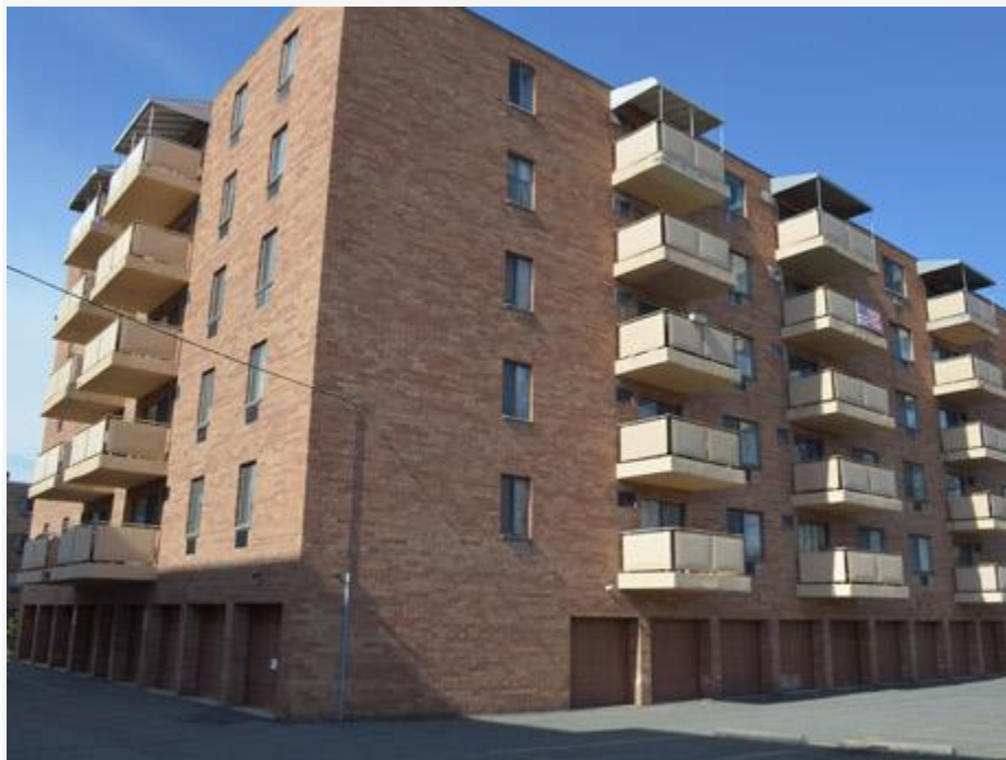
Located at 240 Anderson St., El Dorado Apartments features 53 residential units.
